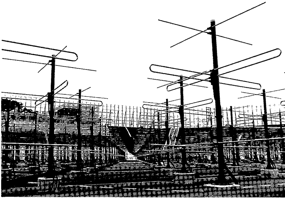
Fig. 4. Photograph taken in the antenna field, showing crossed three-subelement yagis and RF cables.
